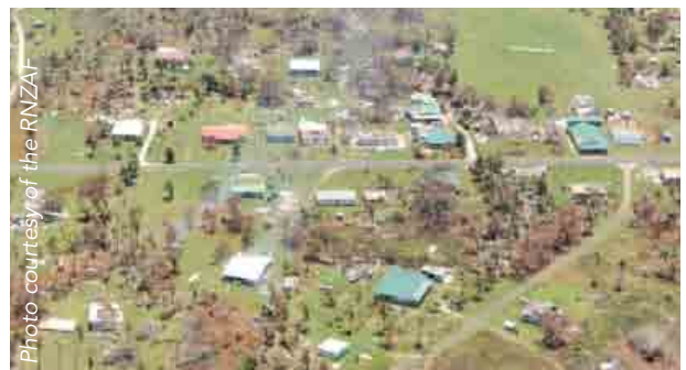
Figure 2: Differing degrees of building damage in Tropical Cyclone Pat in 2010.
